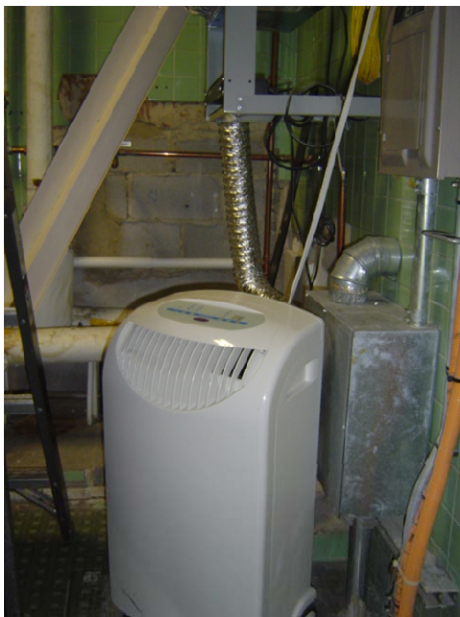
Figure 3.10 Spot Coolers in Former Restroom Reconfigured as Communication Room.
