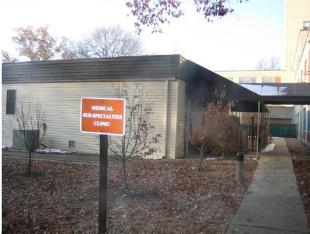
Figure 3.25 Example of a $750,000 “Wart” which is characteristic of the restrictive nature of the current COC funding limits to long range, cost effective facility solutions
