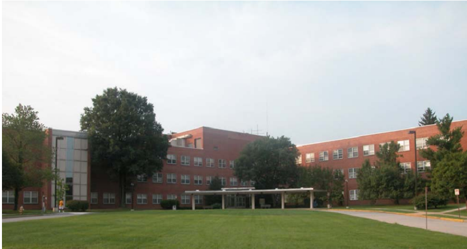
Figure 2.3 Kimbrough Ambulatory Care Center, Fort Meade, Maryland
