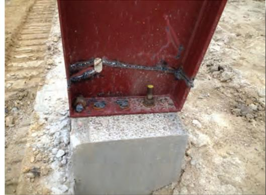
On July 21, 2013, the defendants used an acetylene torch to burn through the steel support columns in a building in retaliation for the contractors' failure to hire union ironworkers.
