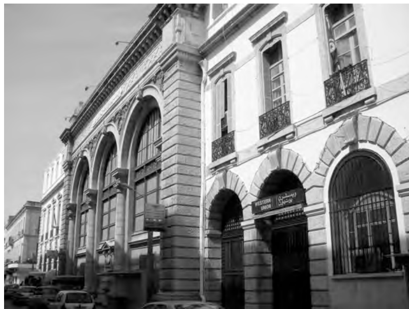
Figure 3.28. 1893 Postal headquarters, Tunis. Henri Saladin, architect. Photograph (2006). (Source: Author's collection.)
