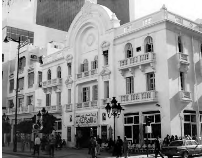
Figure 5.14. Rossini Palace cinema following 2000–2001 restoration. Photograph (2005). (Source: McGuinness et al., Tunis , 46.)
