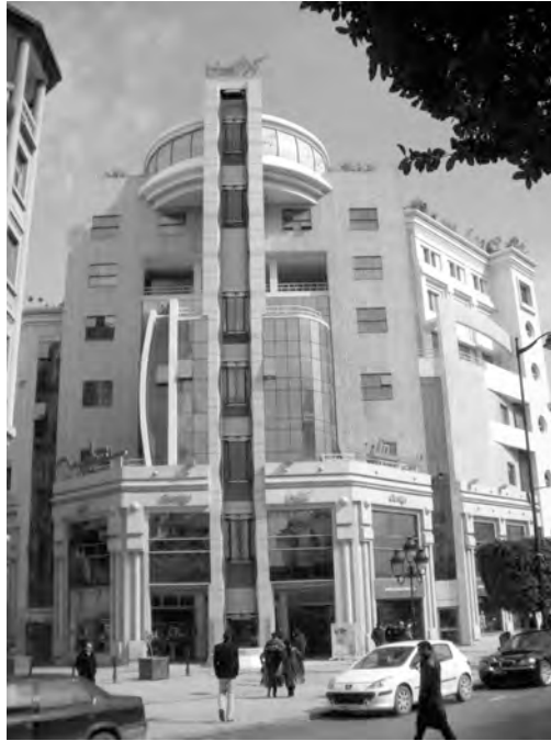
Figure 5.17. The new Claridge Building, Avenue Bourguiba, Tunis. Photograph (2009). (Source: Author's collection.)
