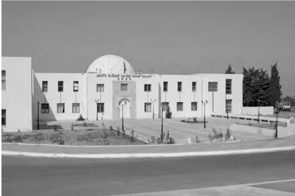
Figure 5.45. ENAU, Tunis. Principal façade. Photograph (ca. 2000). (Source: “ENAU,” Groupe Studi, < http://www.studi.com.tn/site/publish/images/image_gallerie/4_cons/Education/max/enau.jpg >.)
