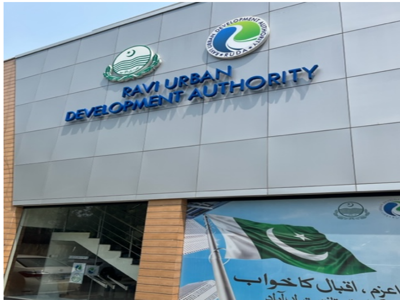
Image 2 The main building of the Authority's Office 3
