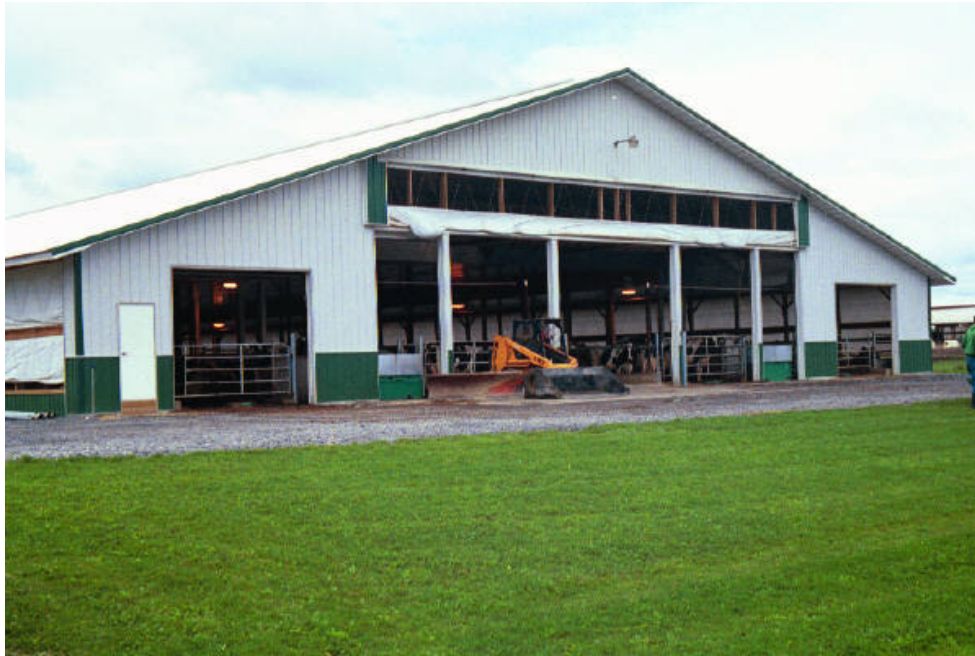
Figure 2. Inlet for a Tunnel Ventilated Six Row Freestall Barn.
