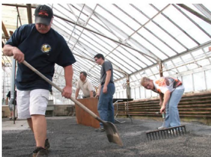
B&P crew laid gravel on the floor of one of the greenhouses to prepare it for use as an exhibit area.
