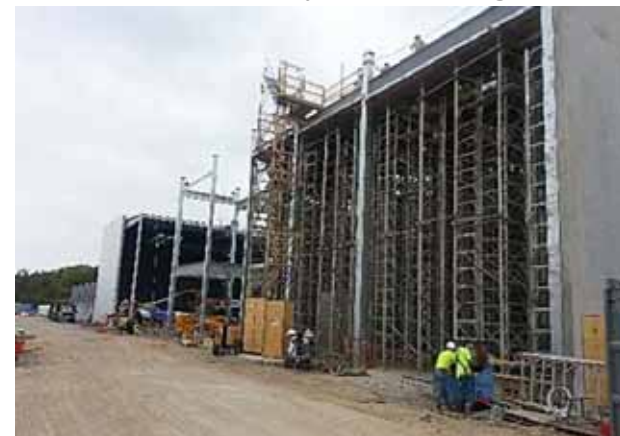
Getting Ready to Pour the 40 foot level of the dryer building
