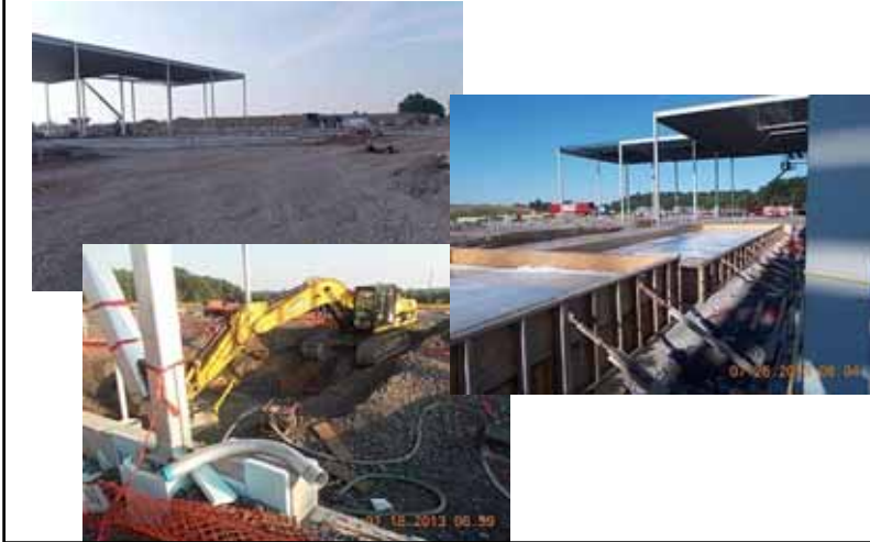
Progress Continued though
