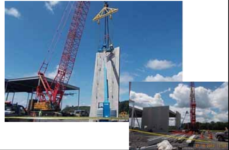
The 300 Ton Crane at Work
