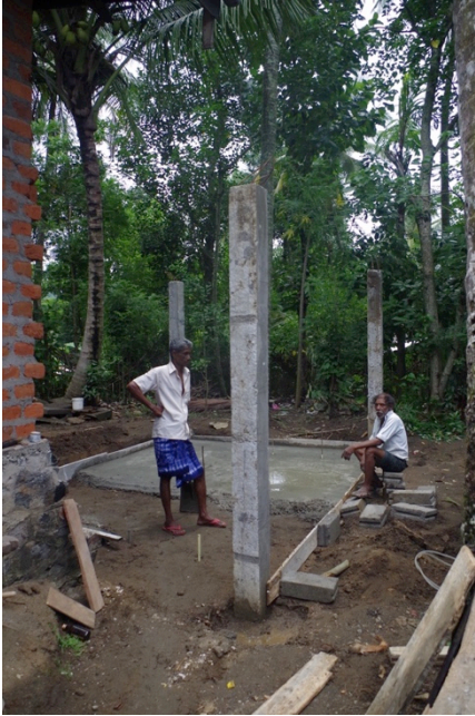
Figure 13-The construction of a work hut in Atwaedagama
