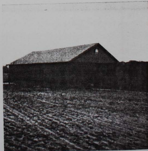
CINDER BLOCK STORAGE Building
