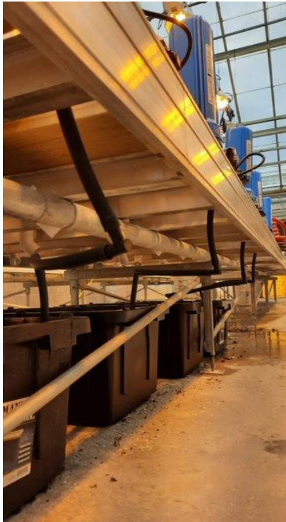
Figure 7. Aeroponic reservoir system. Water is drained from beneath the aeroponic buckets then pumped back up where it is recirculated.
