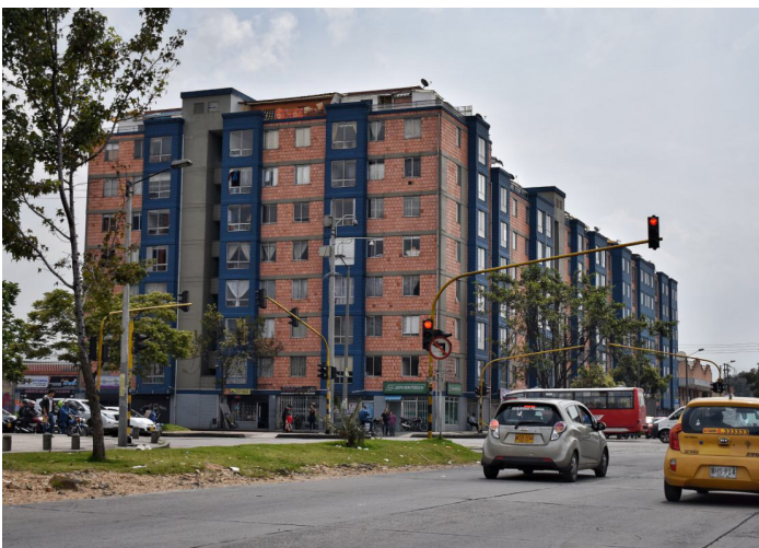
Figure 4: Paloquemao. Example of traditional low-income housing in Bogotá. The free houses offered today resemble this model, normally a five-story walkup building with some space for amenities. Source: Pardo,J. (2018)
