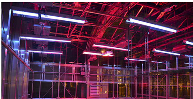
Figure 4. UVB lamps suspended in the superstructure of a greenhouse can suppress powdery mildew on a broad variety of crops with as little as 6 minutes of nighttime exposure twice per week.
