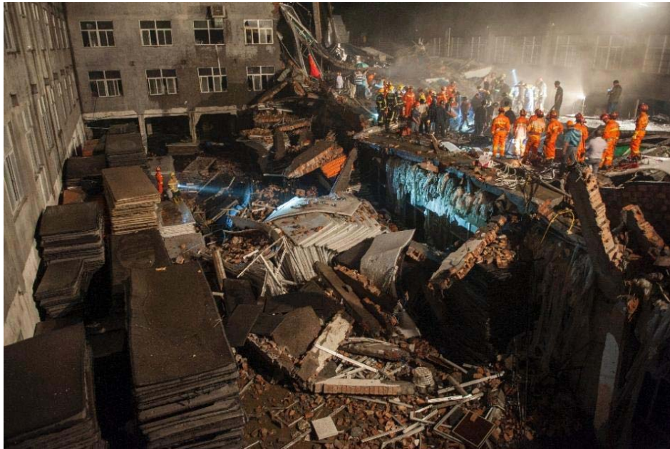
A shoe factory collapsed in eastern China. (Photo credit: AsiaOne ↗ )
