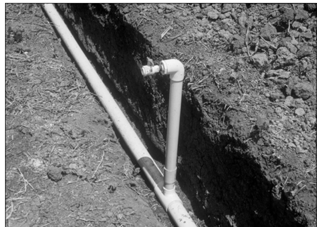
Photo 3-4. PVC pipe trenched in, with riser pipes.
