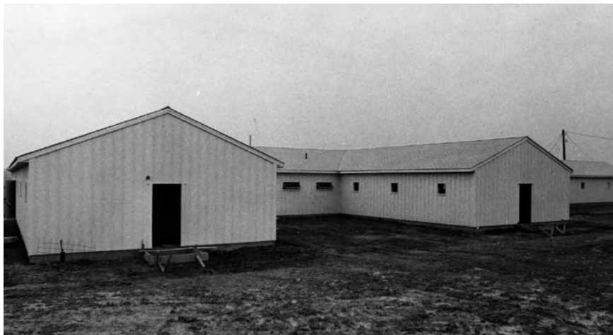
The swine unit on Pine Tree Road nearing completion in 1977
