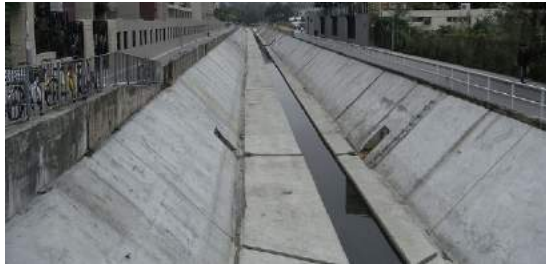
Common nullah in Hong Kong (source: Bladezcafo).
