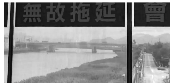
The two-story pedestrian bridge at Lok Ma Chau Station and view on the bridge.
