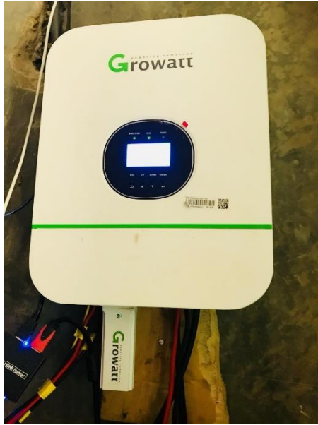
Figure 22: Hybrid Inverter at Vota Ranch Source: Photo provided by Vota Ranch
