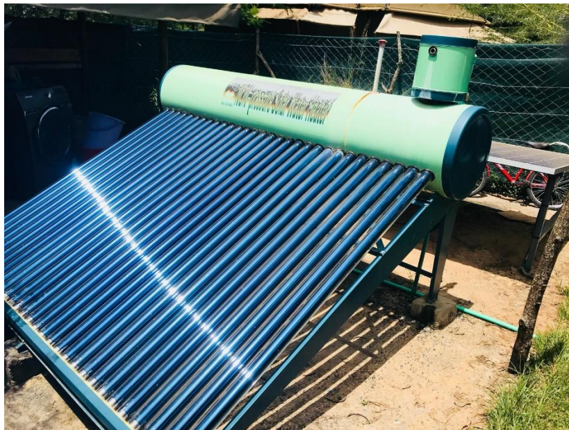
Figure 23: Evacuate Tube Solar Heater at Vota Ranch Source: Photo provided by Vota Ranch
