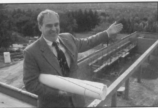
Director Doug Antczak on site at the new laboratory facility for the Baker Institute
