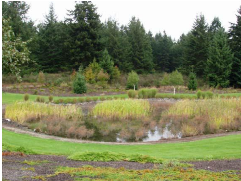
Figure E.2: Infiltration Pond along SR 510 in Thurston County
