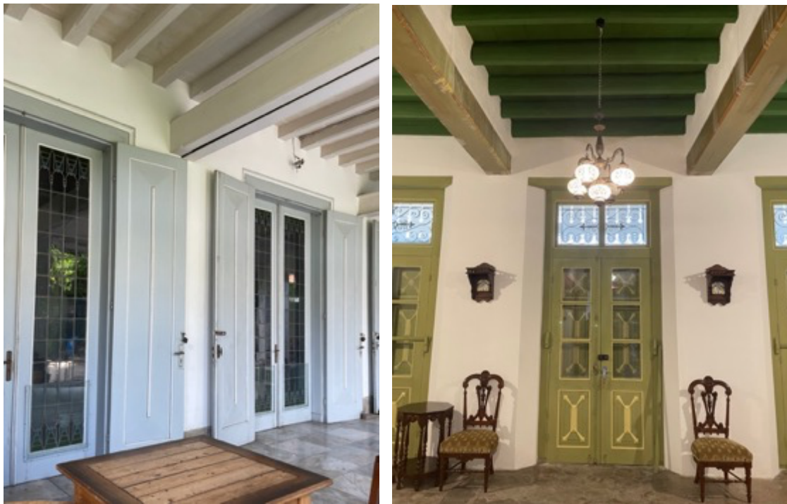
Figure 3.40. Two-leafed Glass Wooden Door at Margo Redjo (left) and Figure 3.41. Two-leafed Glass Wooden Door at The Siek Family House (right) (Source: The Author's Collection)
