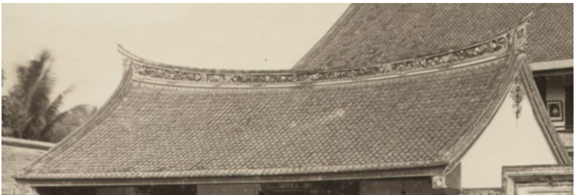
Figure 3.32. The Roof of Candra Naya, which ends with Swallowtails on both ends (Source: KITLV: Woodbury & Page, Batavia)
