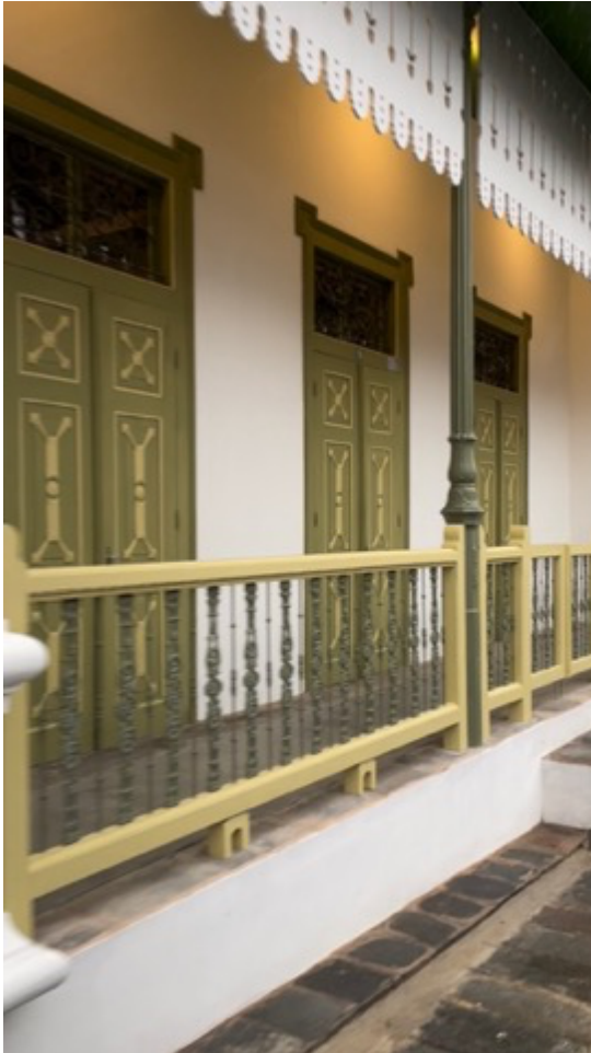
Figure 4.14. The Main Façade of Siek Tjing Liong's House (Source: The Author's Collection)
