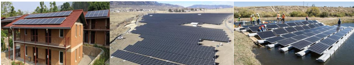
Figure A2: Left - Kopila Valley School in Surkhet, Nepal sites their solar on rooftops to minimize land disturbance. Center - Solar installation on a brownfield site in Colorado. Right - Panels installed on ponds or reservoirs (Sources: author, Kiatreungwattana et al. 2013, and Hernandez et al. 2019, respectively)
