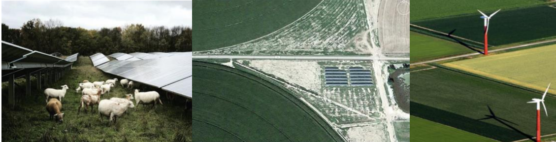
Figure 12: Left - A single plot of land operates simultaneously as a solar facility and grazing land for sheep. Center -Solar panels installed in the unused area of a center-pivot crop field. Right - Wind turbines placed to minimize footprint on agricultural land (Sources: Cornell Small Farms Program, Hernandez et al 2019, Inman 2011, respectively)
