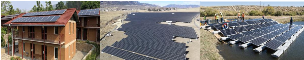
Figure 11: Left - Kopila Valley School in Surkhet, Nepal sites solar panels on rooftops to minimize land disturbance. Center - Solar installation on a brownfield site in Colorado. Right - Panels installed on ponds or reservoirs (Sources: author, National Renewable Energy Lab, Hernandez et al 2019, respectively)
