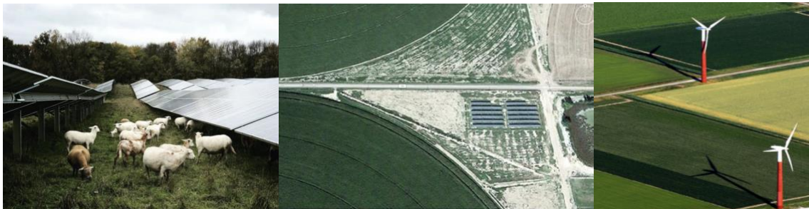
Figure A3: Left - A single plot of land operates simultaneously as a solar facility and grazing land for sheep. Center - Solar panels installed in the unused area of a center-pivot crop field. Right - Wind turbines placed to minimize footprint on agricultural land (Sources: left - Cornell Small Farms Program; center - Hernandez et al 2019; right – Inman 2011)
