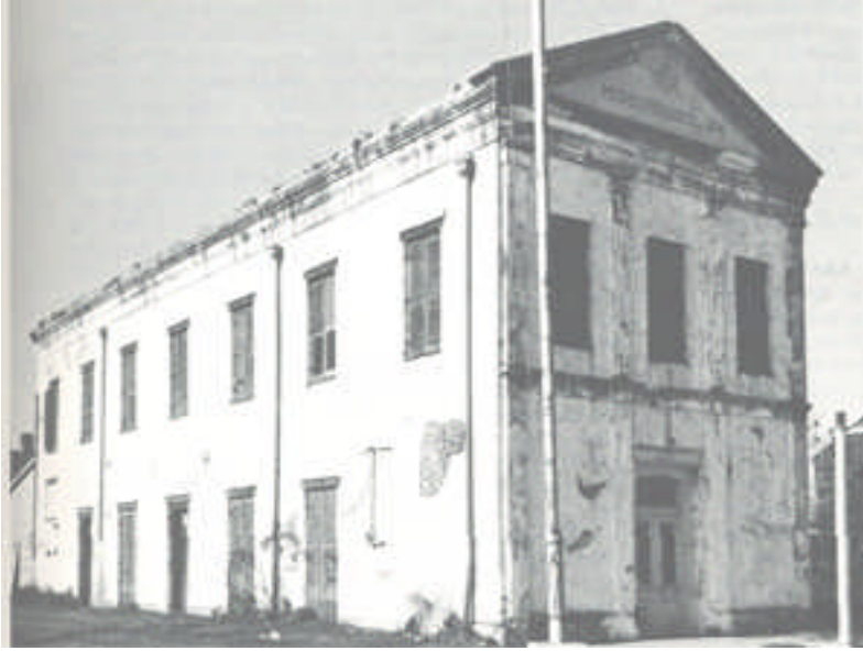
Figure 17: Perseverance Masonic Hall #4 in 1974 in Armstrong Park Christovich, Mary Louise and Roulhac, Toledano New Orleans Architecture Volume VI Faubourg Tremé and the Bayou Road . Pelican Publishing Company: Gretna, 1980: 69.
