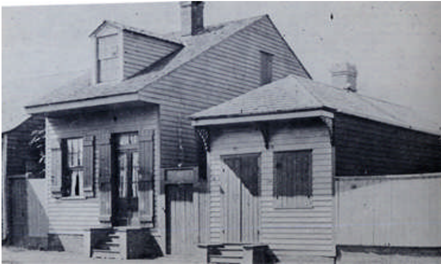
Figure 20: Storyville Cribs. A two-bay Creole cottage and a two-bay shotgun. Christovich, Mary Louise and Roulhac, Toledano. New Orleans Architecture Volume VI Faubourg Tremé and the Bayou Road Pelican Publishing Company: Gretna, 1980:72
