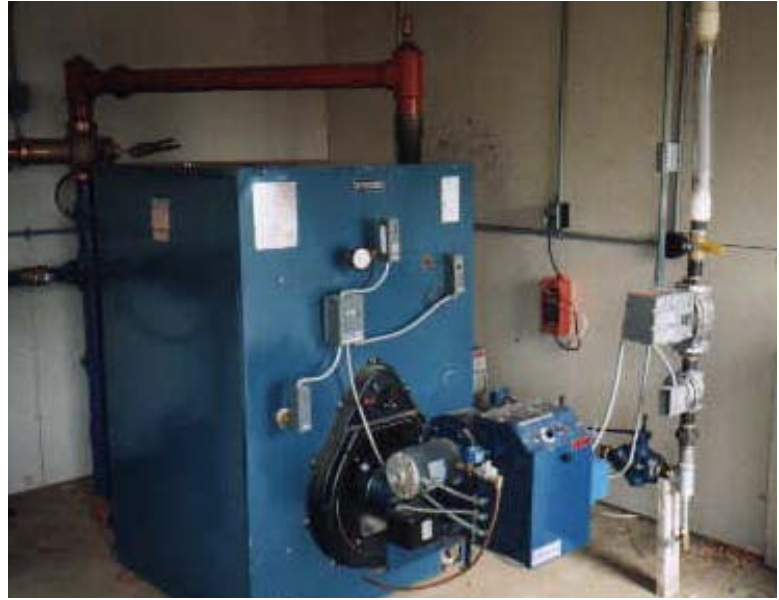
Photo: Moser M, RCM Digesters, Inc.
