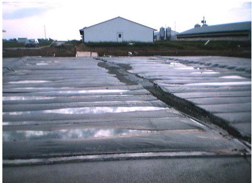
Photo: Moser M, RCM Digesters, Inc.
