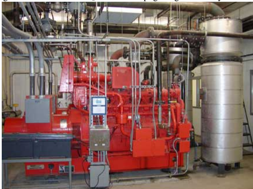
Photo: Ag Environmental Solutions, LLC
