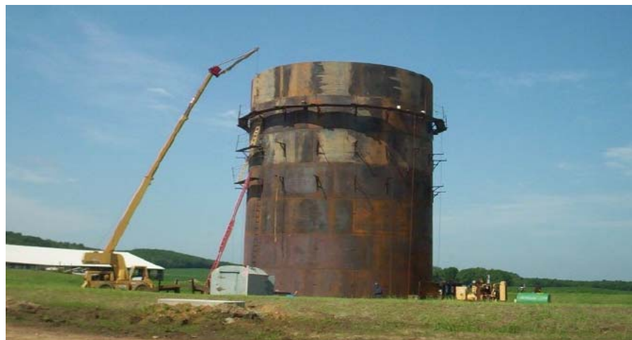
Photo: Eastman D, Microgy Cogeneration Systems
