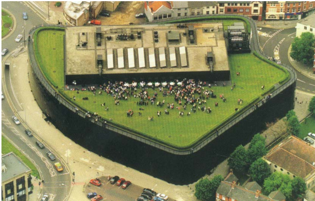
Figure 2.1 - Willis Faber and Dumas Headquarters (Photo credit: Gissen, Big & Green )
