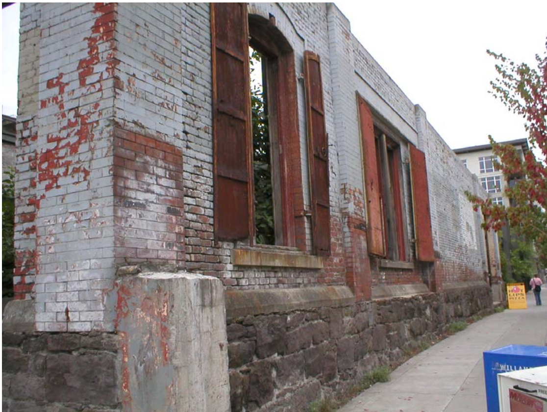
Figure 5.10 - Portion of deconstructed building saved for historic provenance (Photo credit: Author)
