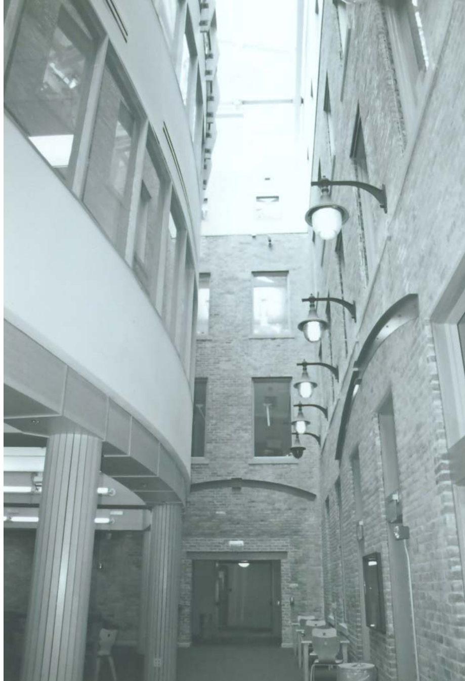
Figure 4.2 - S.T. Dana Building Interior Infill (Photo credit: Author)
