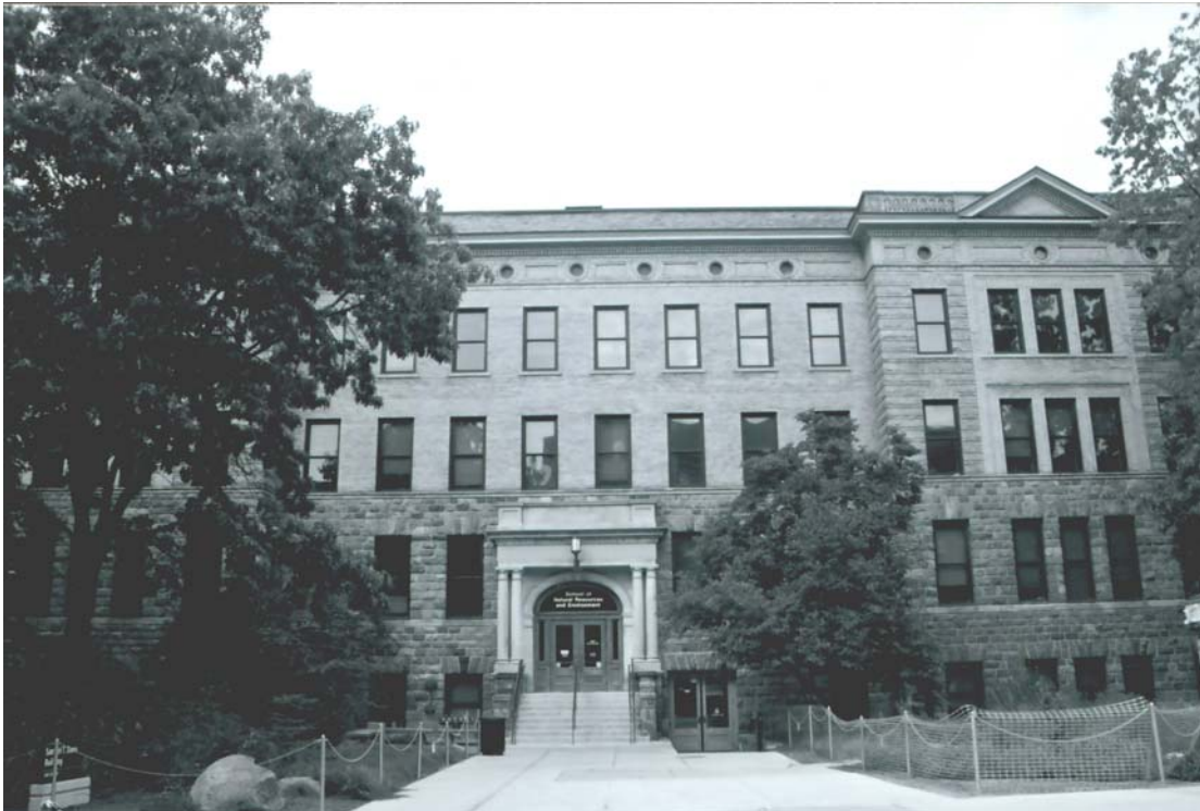
Figure 4.1 - S.T. Dana Building (Photo credit: Author)
