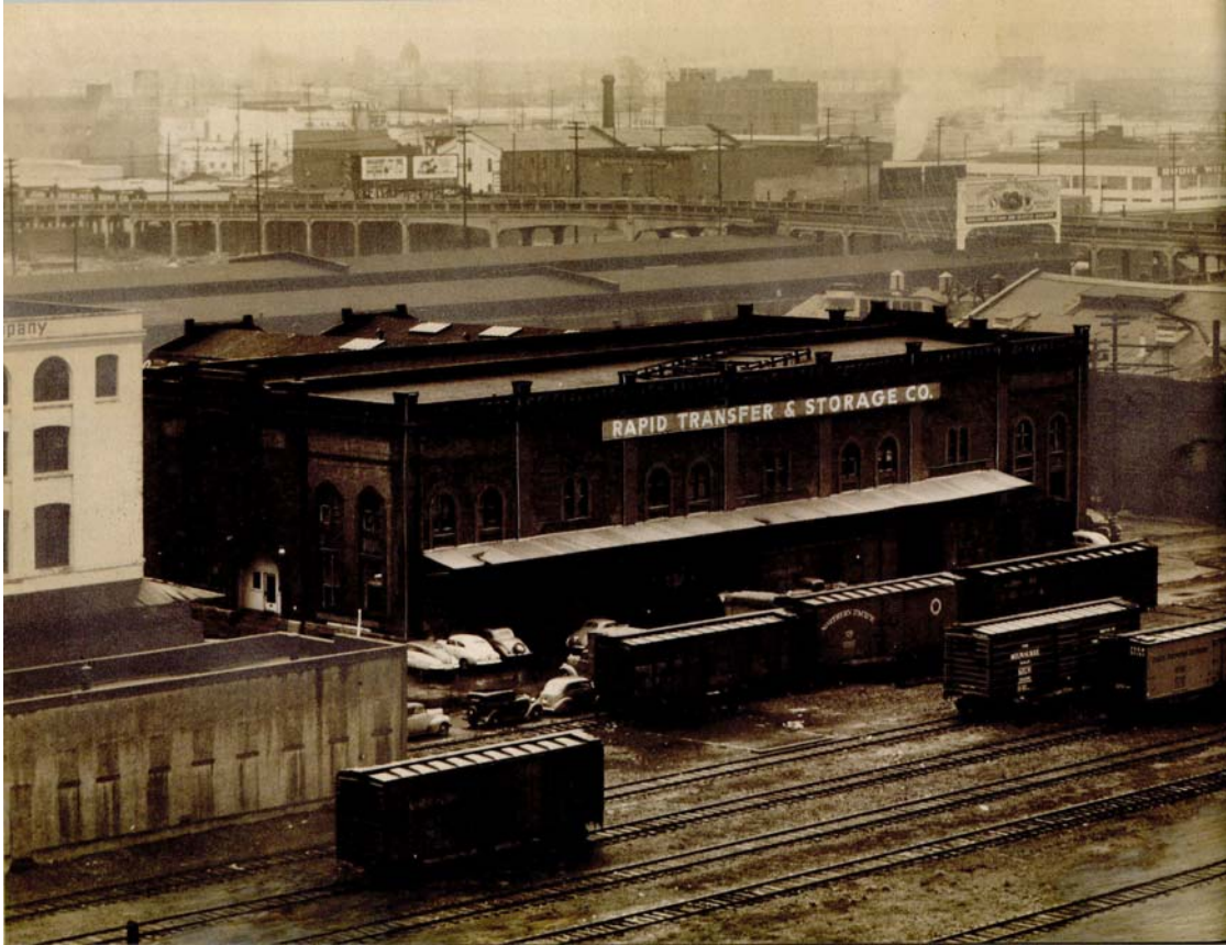
Figure 5.3 - Rapid Transfer & Storage Company (Photo credit: Bettina von Hagen, et al., “Rebuilt Green;” originally from the Oregon Historical Society)
