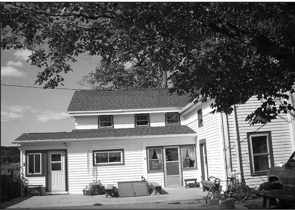
Pratt House, side view.
