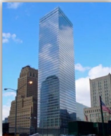
Figure 1: The New 7 World Trade Center Building. Image Courtesy of David Shankbone
