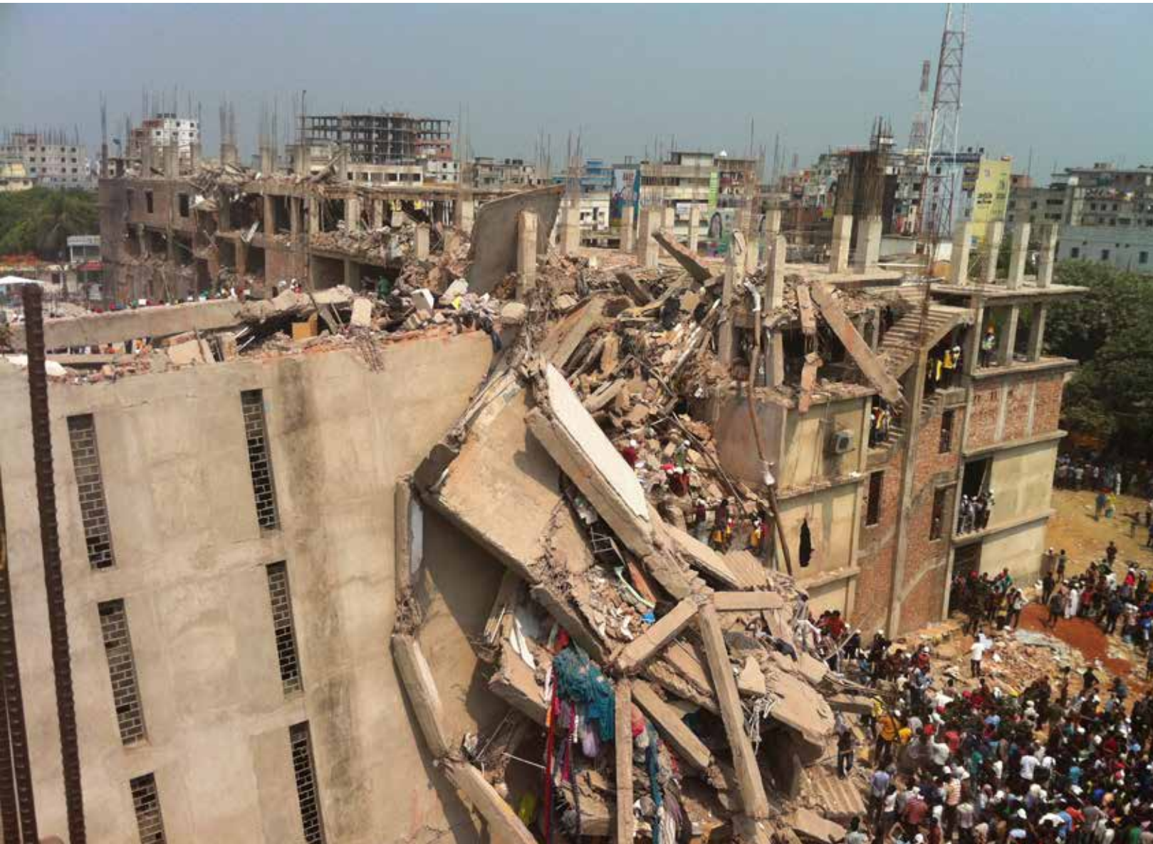
Rana Plaza building collapse, April 24, 2013. © Laura Gutierrez
