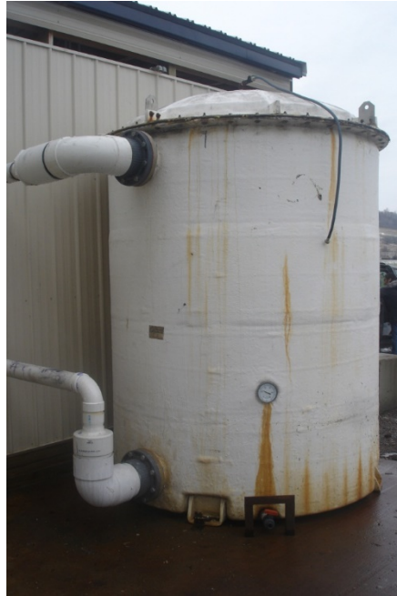
Figure 13. Iron sponge biogas clean-up system on a central NYS dairy farm AD system (Source: C. Gooch).
