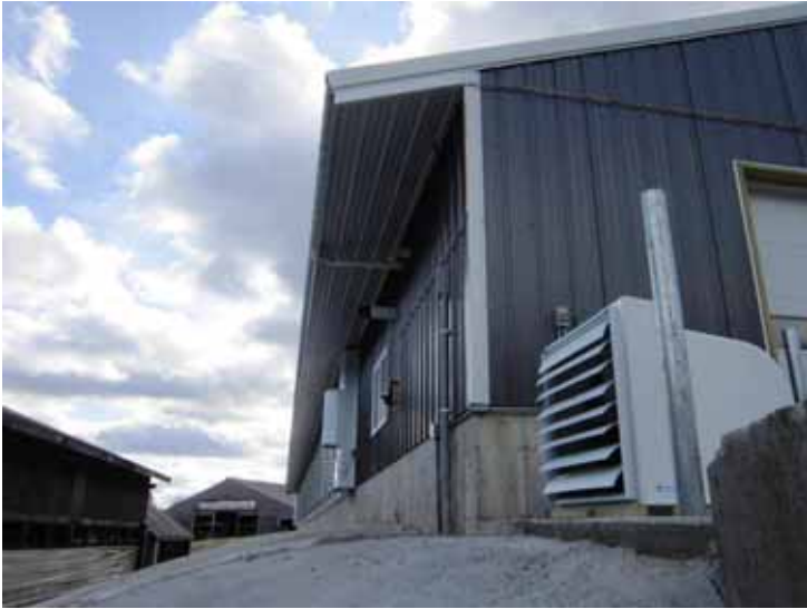
Exhaust plenum fans
