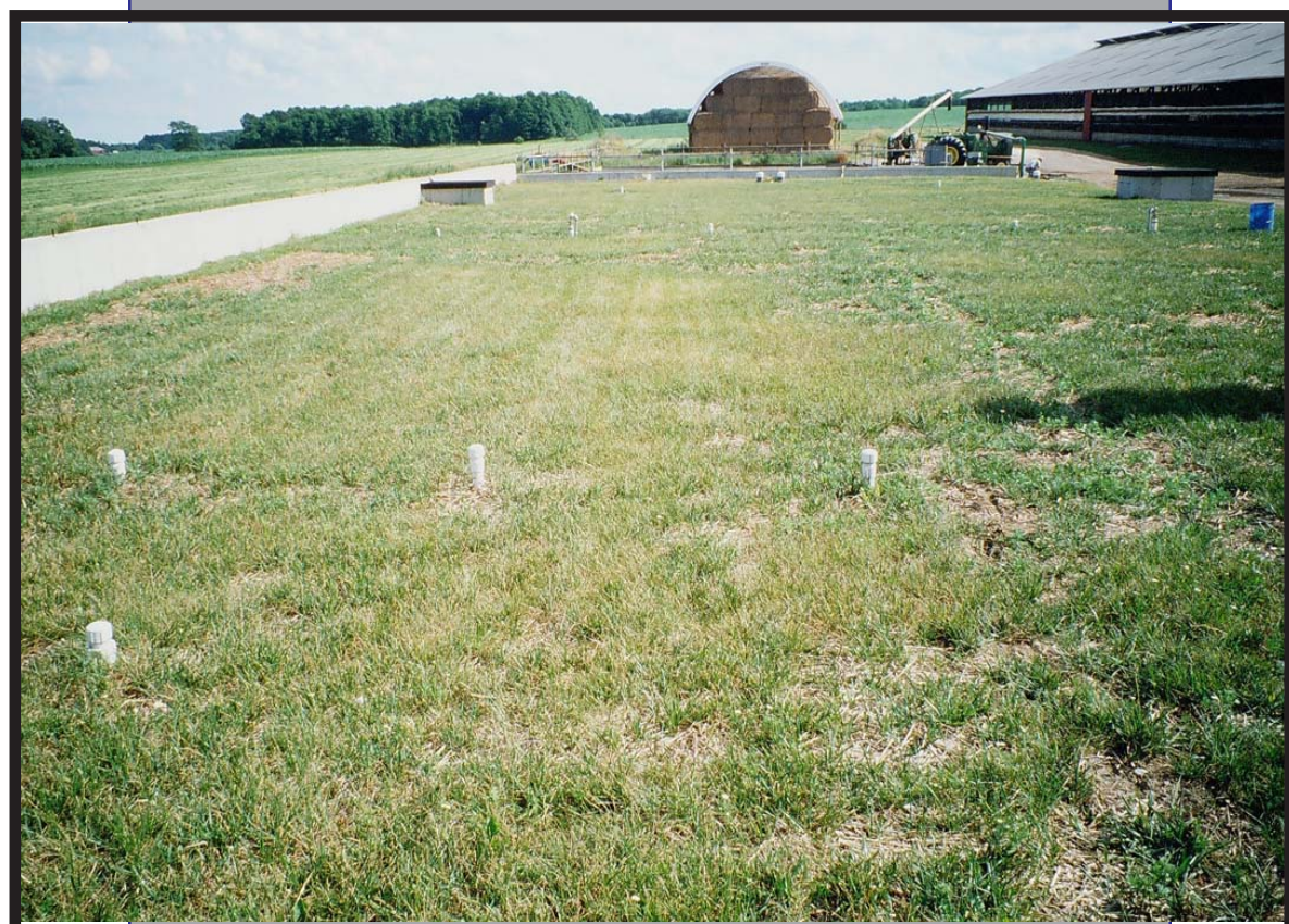
Noblehurst hard-top plug-flow digester (located beneath sod layer)
