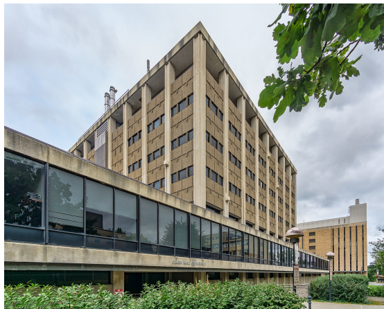
Figure 2: CCMR at Clark Hall
