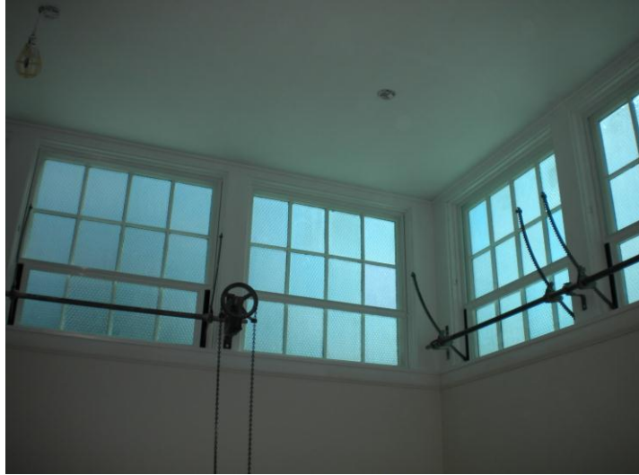
Illustration 12: Original Clerestory Windows in Monitor. (Source: Personal photograph by author. 3 Mar. 2012)
