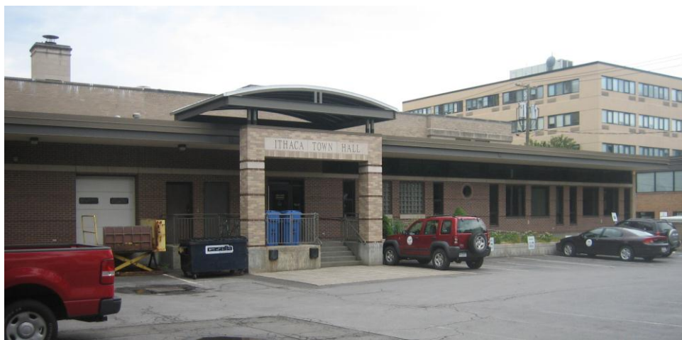
Illustration 8: View of Enclosed Loading Dock. (Source: Personal photograph by author. 25 July 2012)
