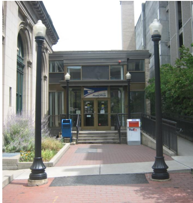
Illustration 10: Glass and Aluminum Entry Vestibule for Postal Store. (Source: Personal photograph by author. 25 July 2012)
