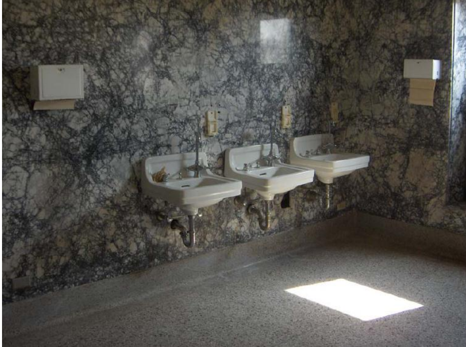
Illustration 23: Photograph of the Marble Wainscot in the Men's Restroom. (Source: Historic Resource Report . Christopher A. Joseph & Associates. Oct. 2007)
