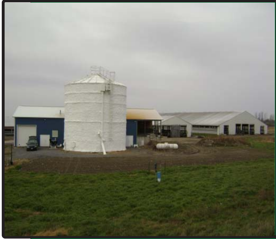
Vertical complete-mix digester with engine building in background
