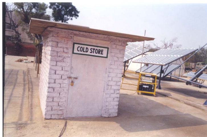
Plate 2. Solar photovoltaic powered cooling system for potato storage.
