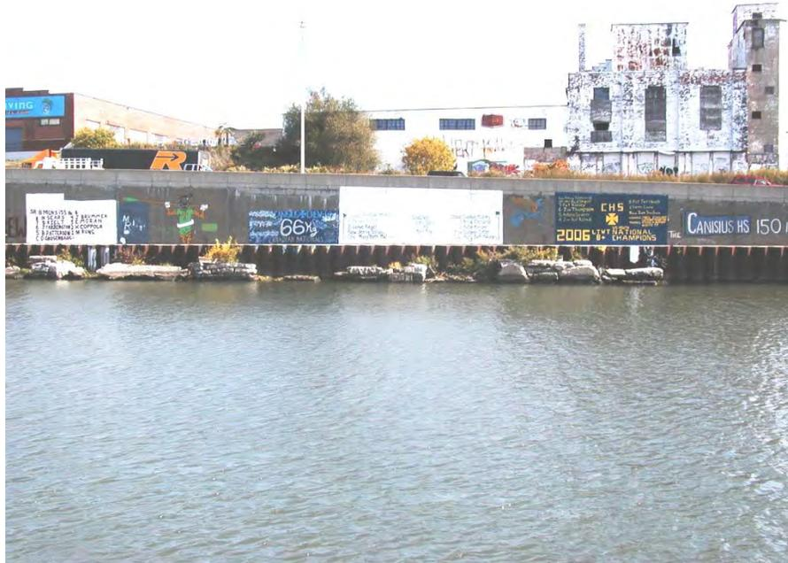
**Stacked Stone Retaining Wall and Sheet Piling South of W. Ferry Street Draw Bridge.
