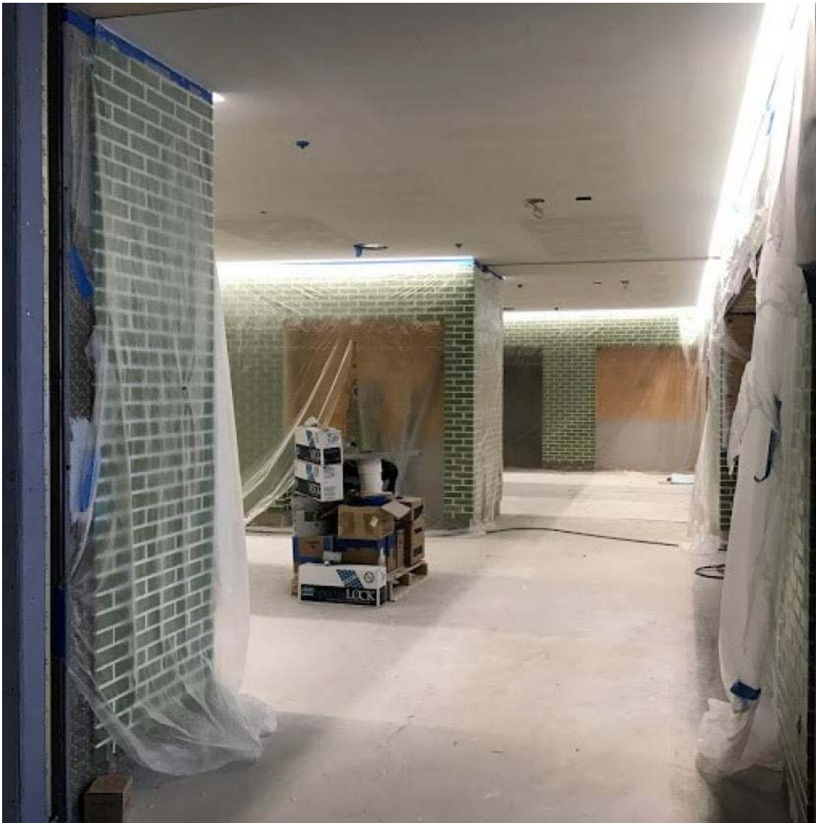
Tile work in new cafeteria area
