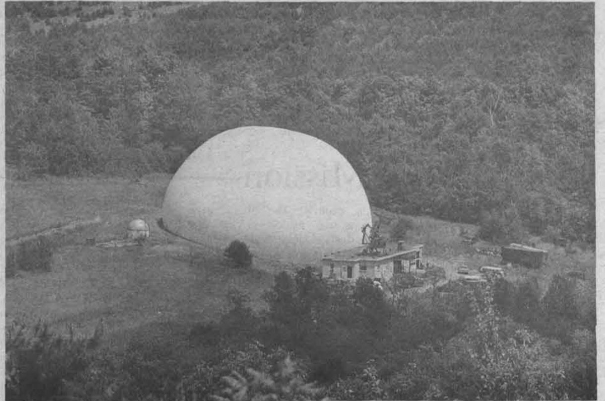
Another part of the NAIC is the radio telescope at the Danby Observatory not far from the Cornell campus. It too is being upgraded. This spring a vinyl coated nylon cover was blown up over the reflector dish to protect the surface from the winter ice and snow and the dramatic daily changes of temperature.
