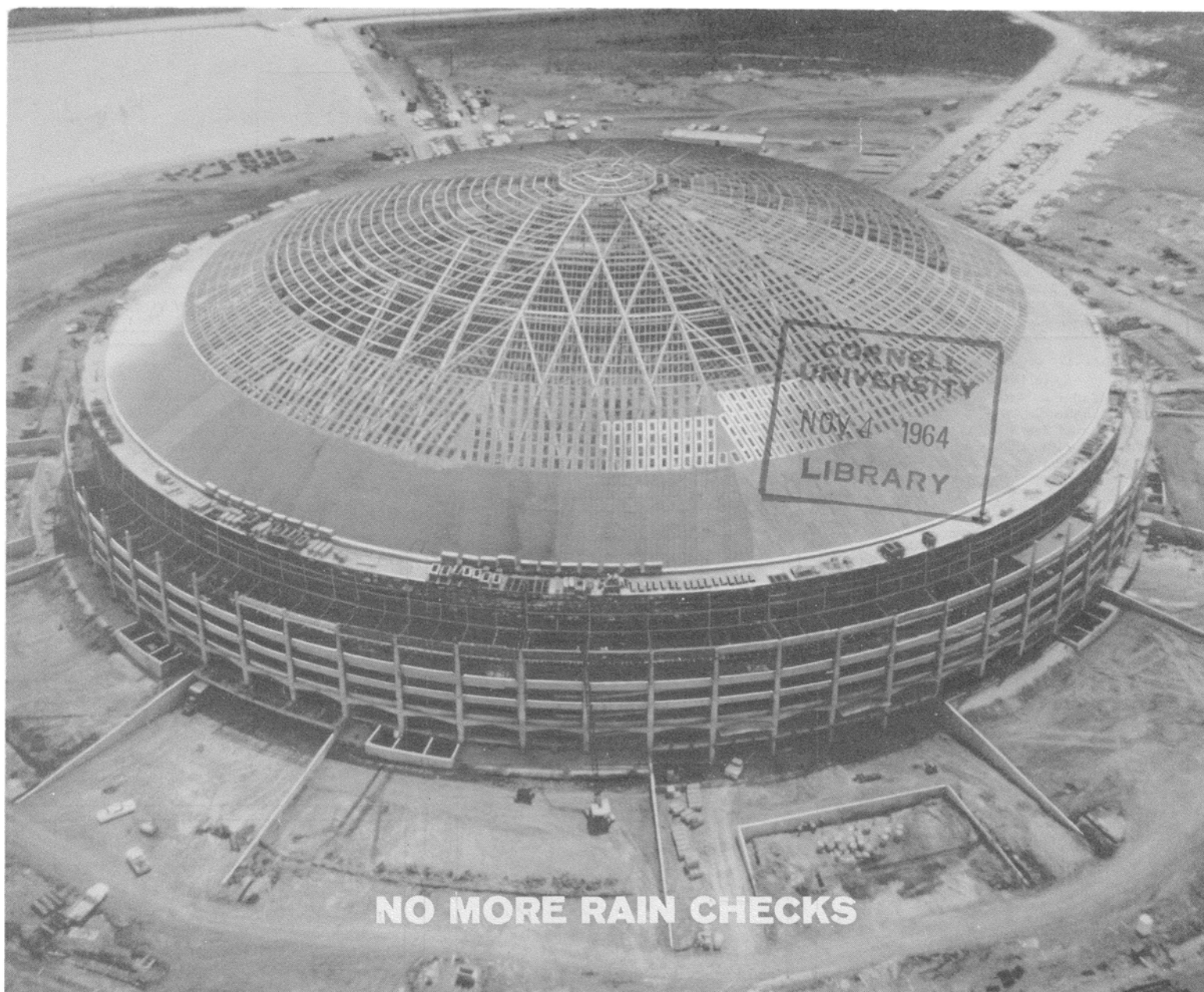
Harris County Domed Stadium, now under construction in Houston, is roofed with panels combining transparent and translucent plastic, and panels of acoustical fiberboard over a steel frame
