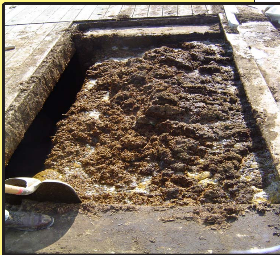
Effluent pit with undigestable bedding solids build-up
