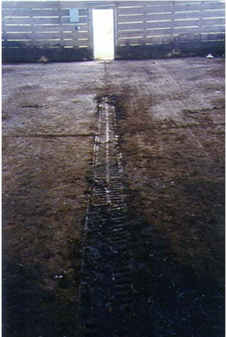
*Impervious compost pads with run-off control provisions for controlling leachate.*
