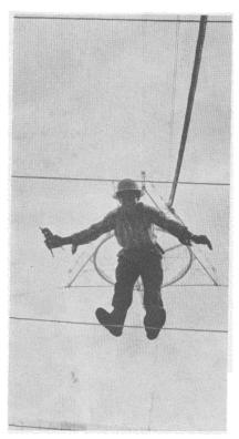
Worker attaches reflector mesh to cables.
