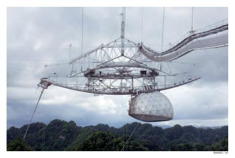
Wide array: Instruments are suspended 150 meters above the dish by wires connected to three towers. Upgrades include a Gregorian dome, added in 1997, which focuses radio signals.
