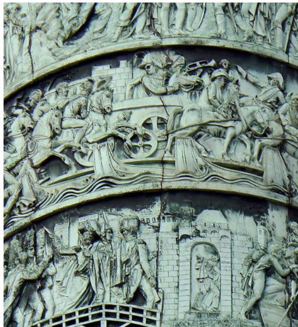
Figure 1.39. Detail of the narrative band on the Vendôme Column , where cracks are visible. (Wikimedia Commons/MBZT, 2011).
