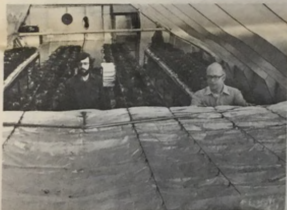
Insulated blanket conserves heat in commercial greenhouses.
