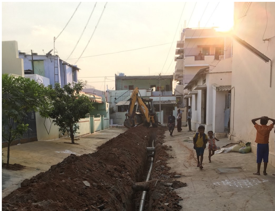
Figure 3.6 - Installation of a new distribution system for the 'Fourth Scheme'
