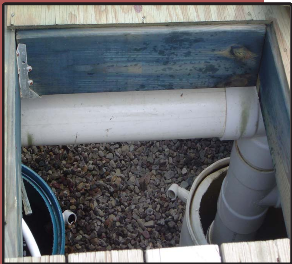
Water column levels in these buckets regulate the maximum biogas pressure
