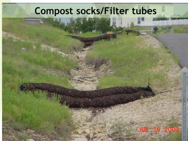
Compost socks reduce sediment, fertilizers, chemicals, metals and other pollutants from reaching surface water by acting as a filter.
