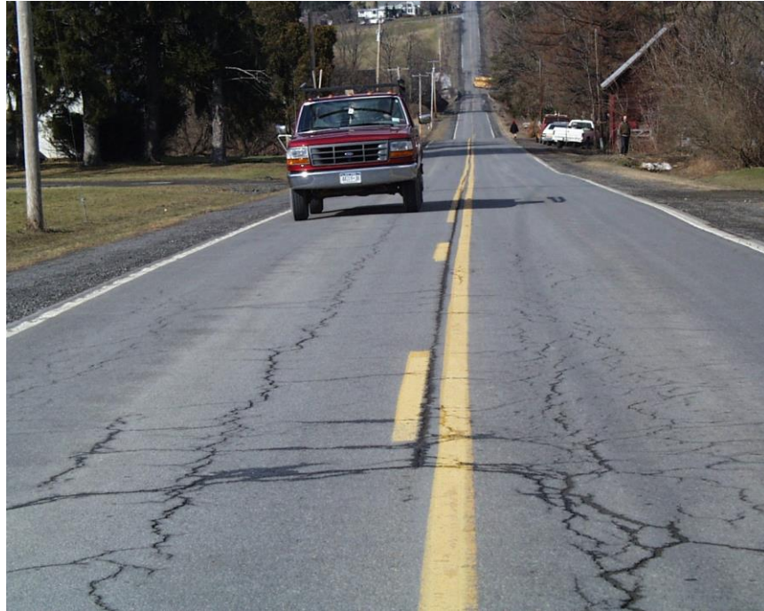
Figure 5 Frost heave cracking (in wheel path) and construction joint crack (on centerline)
