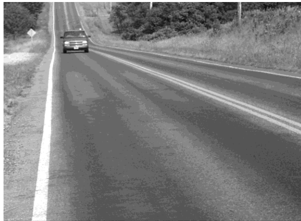
Figure 30 Bleeding asphalt
