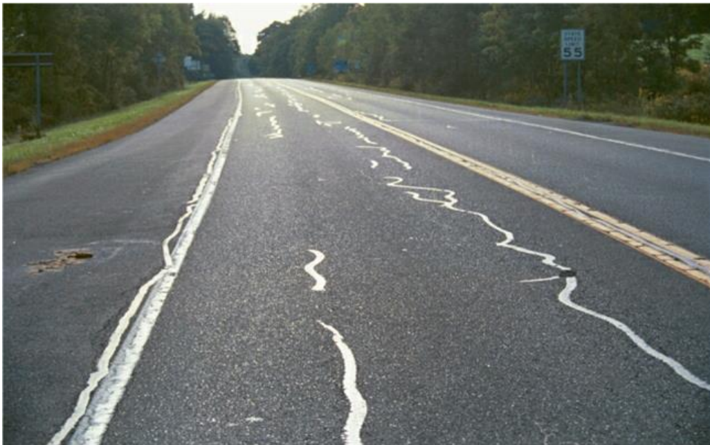
Figure 23 Longitudinal wheel path cracking
