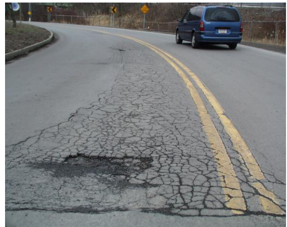
Figure 20 Alligator cracks with pothole
