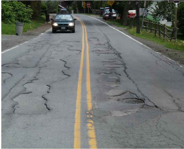
Figure 28 Delamination of an overlay
