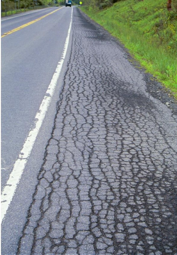
Figure 19 Alligator cracked shoulder
