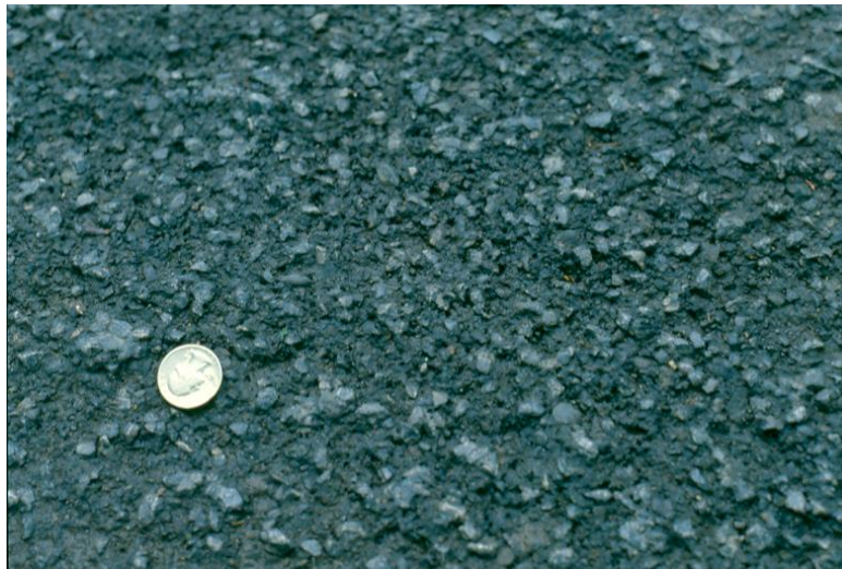
Figure 27 Surface raveling of an asphalt pavement
