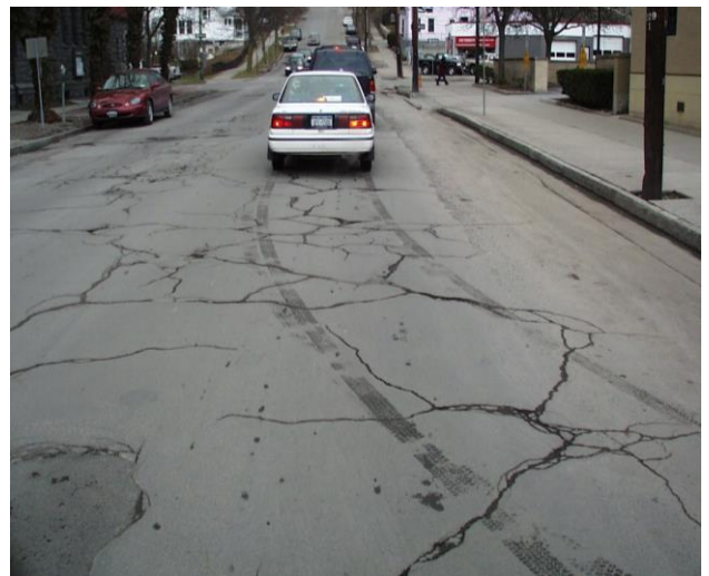
Figure 22 Block cracking
