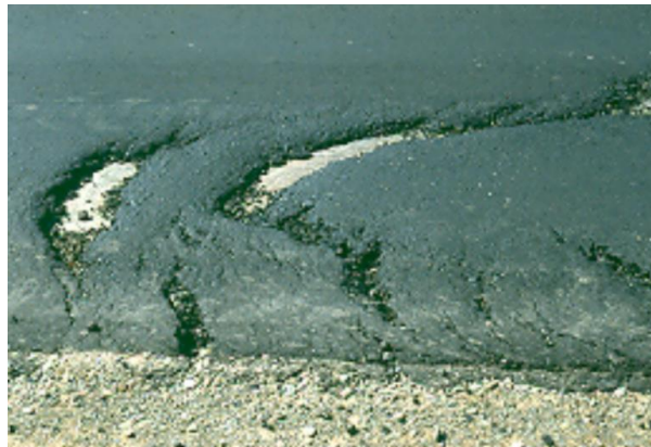
Figure 25 Slippage cracks
