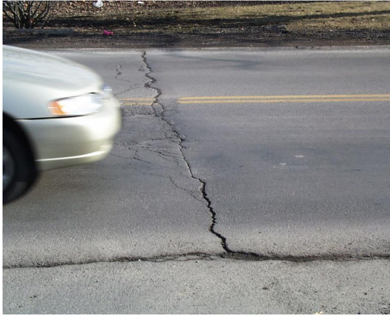
Figure 21 Thermal/low temperature cracking
