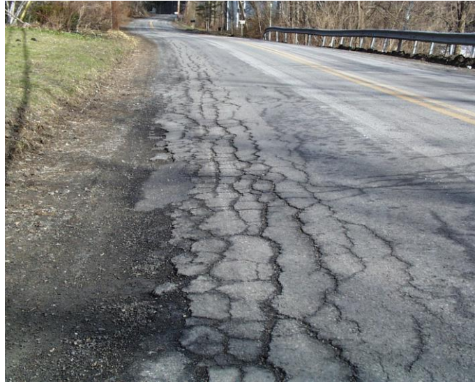
Figure 24 Edge cracks
