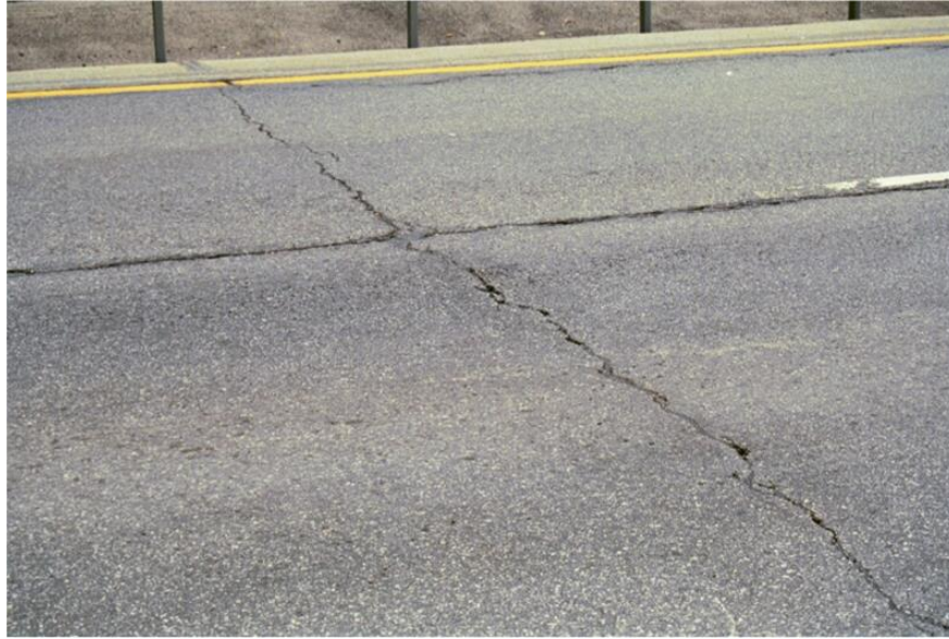
Figure 18 Reflective cracks in an overlay
