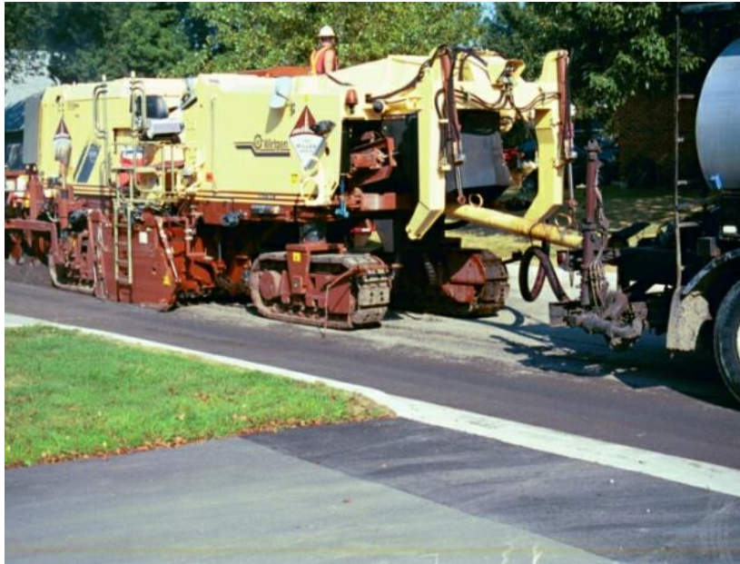
Figure 33 Single unit half-lane recycling train
