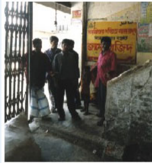
The main stairway from where the workers tried to escape but found the gate locked. The force of people broke down part of the railing.
