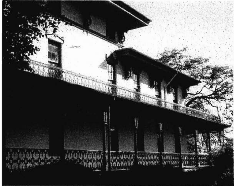
Figure 2: West elevation showing the wing to the rear of the main block. View from the northwest.
