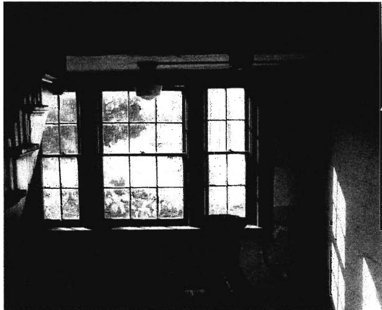
Figure 8: View of landing between first and second floors showing three-part window.
