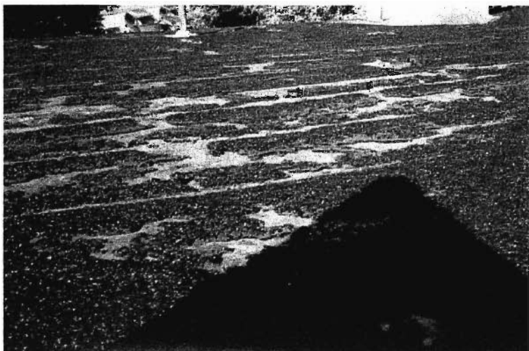
Figure 5: Roof of main block. View towards the west/northwest.
