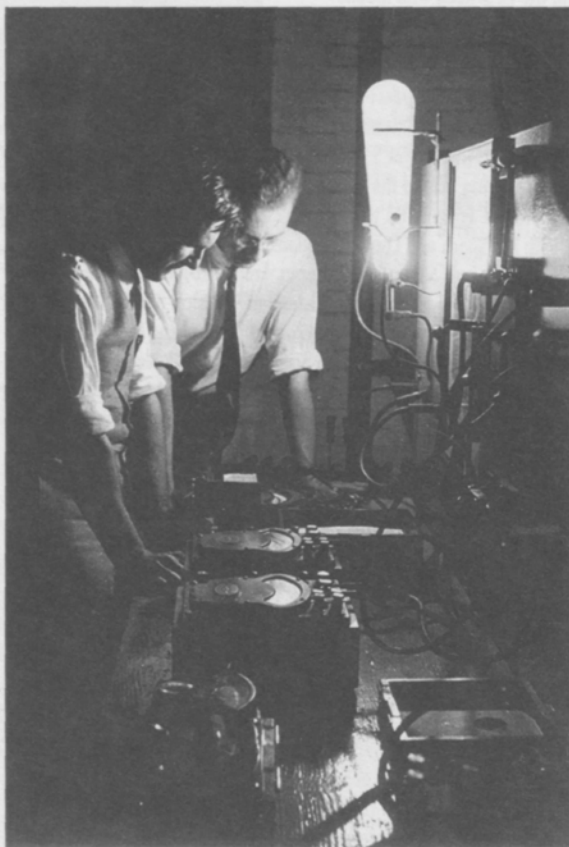
Above, Figure B. Professor Paul Ankrum's electronic regulator for the dc generator. The two glass tubes are grid-controlled mercury-vapor thyratrons in a full-wave rectifier circuit.
